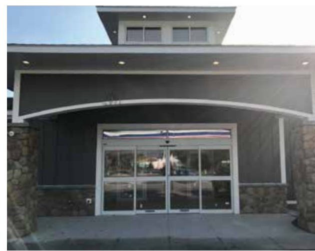
PHOTO | The EZ Market in Onekama will be fully open for the 2018 season. The property has been completely rehabilitated with new gas pumps, all new deli, wine, beer and artisan foods in addition to all of your convenience favorites.
